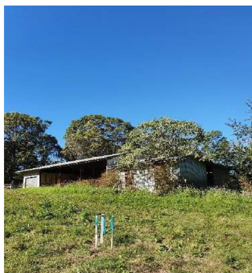
P2 – Shed structure surrounded by fencing
